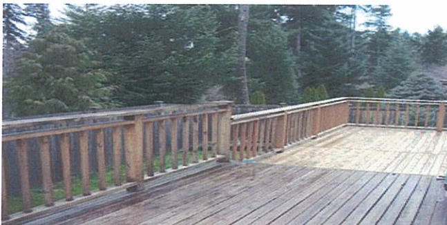
Figure B Deck with Railing
